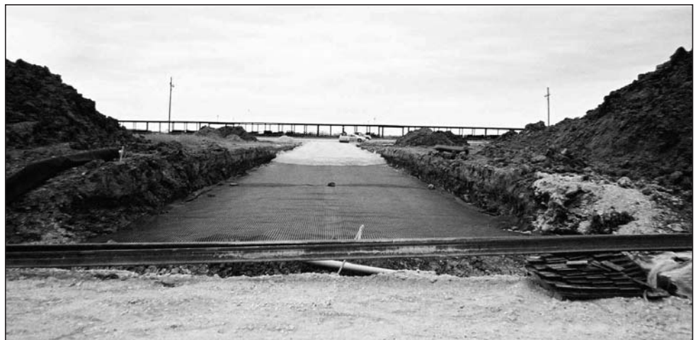
Figure 3. BX1200 Geogrid is used for subgrade improvement on this access roadway to a new facility being built across railroad tracks.
