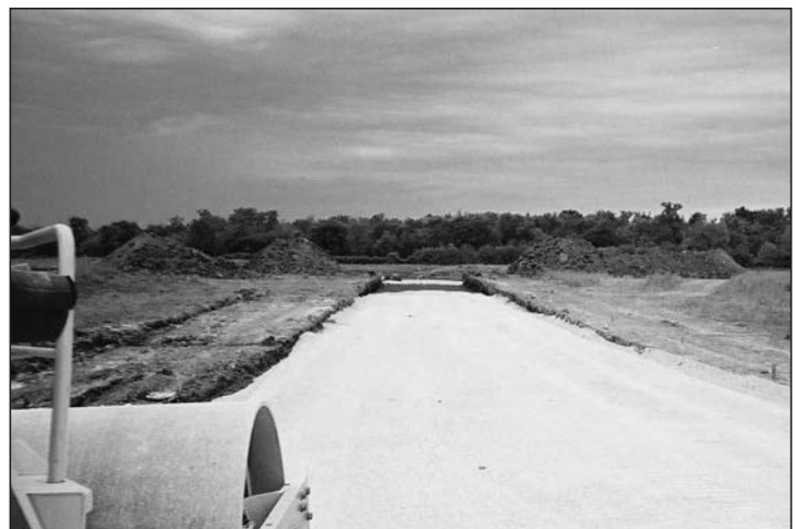
Figure 5. During the base course placement and compaction phases, BX1200 Geogrids prevent rutting from developing.
