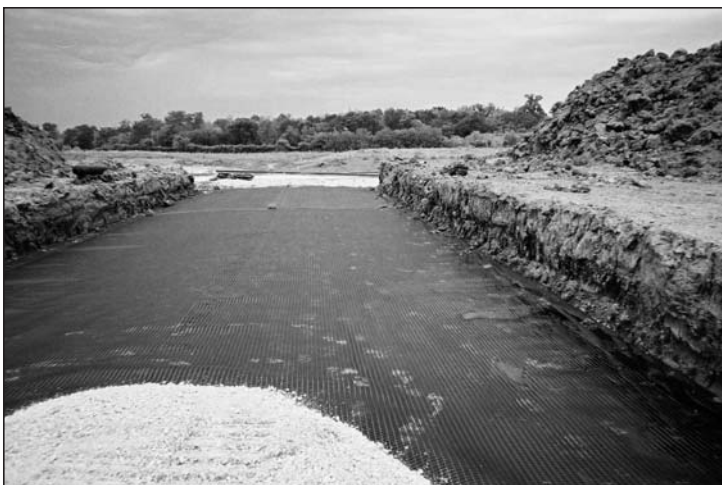
Figure 4. The correct placement of the fill on top of the BX1200 Geogrid is shown as it is placed along the center lap and spread to the edges to minimize any shifting of the geogrid.
