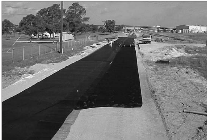
Figure 2. The ease of installation of BX1200 Geogrid helped the construction crew stay ahead of the fill operations.
