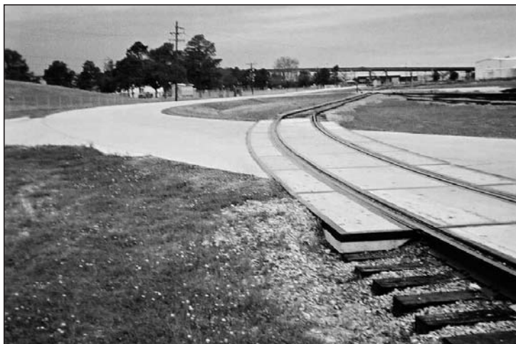
Figure 6. The finished Ernest Wilson Drive roadway at the railroad crossing where BX1200 was used beneath the base course.
