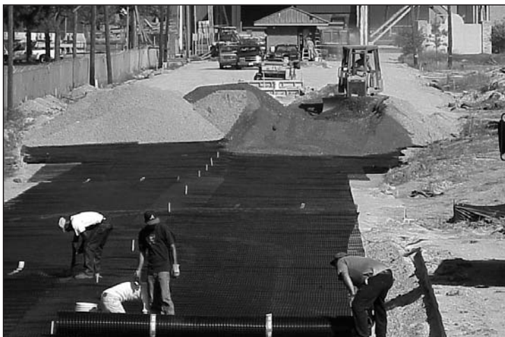
Figure 1. Initial placement of limestone base course is being made on top of the BX1200 geogrid for the Ernest Wilson Drive reconstruction.
