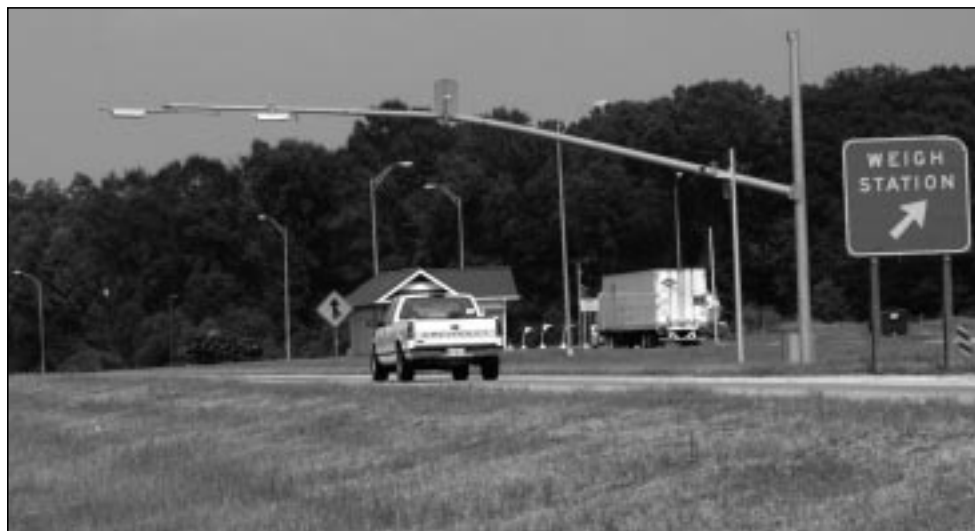
Figure 5. This view of the third technology gauntlet from the median shows from the left the compliance AVI antennae and the wireless communication antenna cantilevered over the roadway, and a pole-mounted closed circuit television camera.
