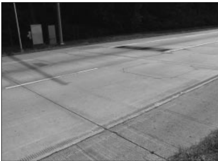
Figure 8. A broader view from the median and downstream showing the WIM scale and various inductive loop sensors cut in the pavement and a piezoelectric sensor located downstream of the WIM scale.
