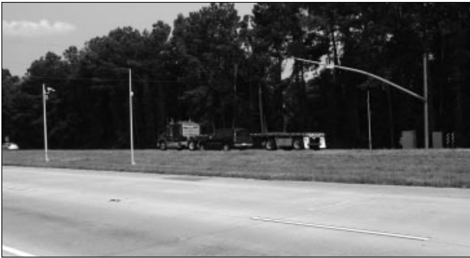
Figure 3. This view of the first technology gauntlet from the shoulder of the opposing roadway shows from the left pole-mounted closed circuit television cameras, the over height vehicle detector
