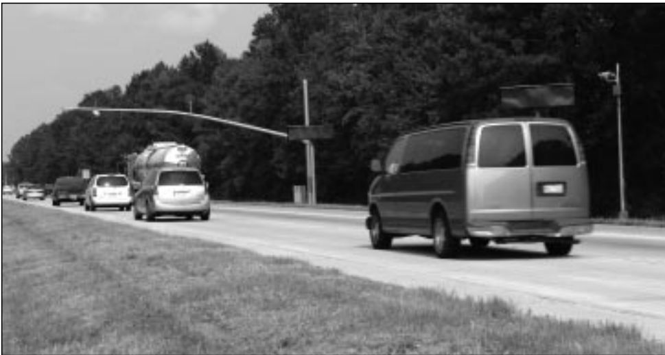
Figure 4. This view of the second technology gauntlet from the median shows from the left the incab notification antenna and wireless communication antenna cantilevered over the roadway, 2 pole-mounted changeable message signs, and a pole-mounted closed circuit television camera.
