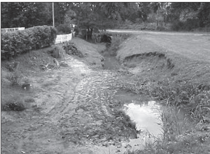
Figure 9. (Above) Channel erosion in an open drainage ditch.
