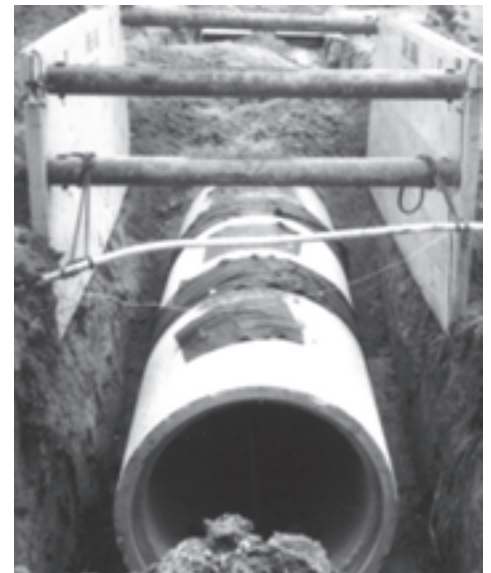
Figure 12. Storm sewers ostensibly alleviate all problems associated with channel instability by totally enclosing the flow.
