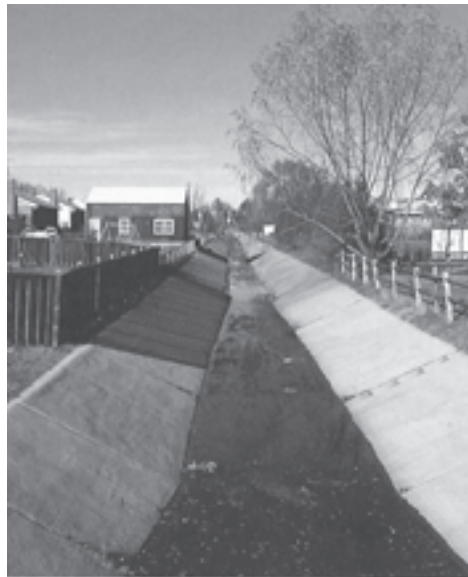
Figure 11. Armoring a channel with concrete liner to prevent erosion.
