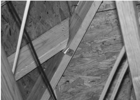
Figure 6. Rafter connection made to the sheathing at a roof hip. Straps should also be connected to the valley sheathing
