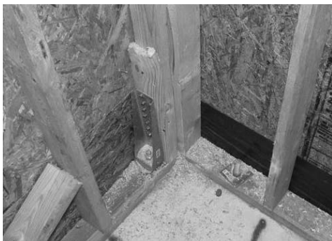
Figure 13. Corner conditions can require a more substantial hold down as in this example where a Simpson hold down device attached to the corner studs is used in lieu of threaded rods located near the corner and anchoring the top plate.
