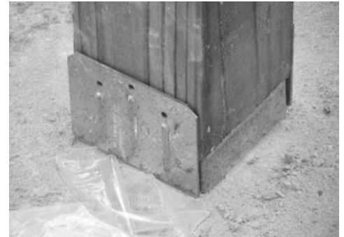
Figure 18. This corner post receptacle equipped with dowels that are inserted into holes drilled into the concrete slab. It is glued to the concrete slab with an epoxy and then nailed to the post to resist uplift forces.
