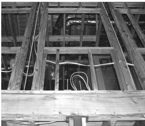
Figure 10. Threaded rods are anchored with square oversized washers recessed into the bottom of a second floor support beam to which they transfer the uplift forces from the top plate of the second floor wall. The rods are located either side of an opening in the second floor stud wall. The uplift forces are transferred through the second floor support beam to the first floor square steel tube column attached to the beam with two threaded rods anchored by oversized square washers located on top of the beam.
