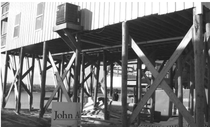
Figure 20. Driven timber piles are extended above the ground line and serve as the columns to support this residence in a flood prone area.
