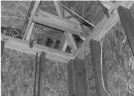
Figure 5. Rafter connection straps to the top wall plate shown in a corner and also shown are two threaded rods anchoring the top plate to the foundation.
