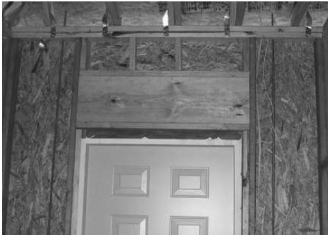
Figure 16. The threaded rods either side of the door opening provide continuity to resist the uplift forces over the door that are transferred by the shear wall also over the door.
