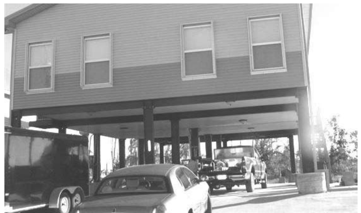
Figure 21. The monolithic foundation slab cast on the ground under this elevated residence provides the support for the open steel frames that support the residence. The columns are anchored to the slab that approximates flexural fixity at their base.
