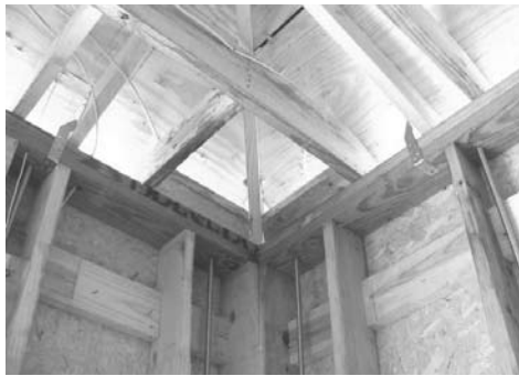
Figure 7. Rafter connection straps to the top wall plate shown in a corner and also shown are 4 threaded rods through the top plate with 3" square oversized washers anchoring the top plate (not shown).
