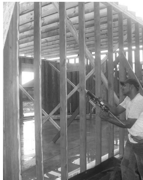
Figure 14. A glue bead is being applied to the studs before attaching the exterior wall sheathing.
