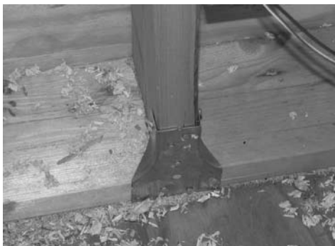
Figure 11. This is an example of an installed alternative connection to the U strap that connects studs to the top and bottom plates.
