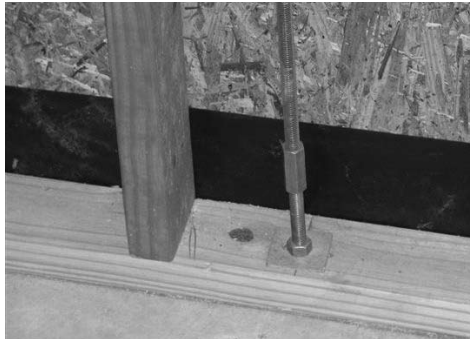
Figure 8. Bottom plate is shown with an anchor bolt equipped with a square, oversized washer and a threaded coupling to extend the threaded rod to anchor the top plate (not shown).
