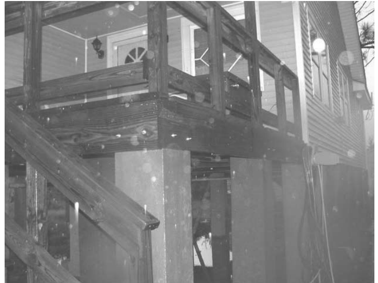
Figure 19. Cast-in-place reinforced concrete piers or columns support this elevated residence in a flood prone area.
