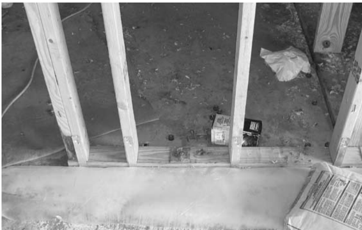
Figure 9. Interior wall hold down unit with anchor bolts in the bottom plate equipped with 3" square oversize washers. U straps connect the studs to the bottom plate and the top plate (not shown).
