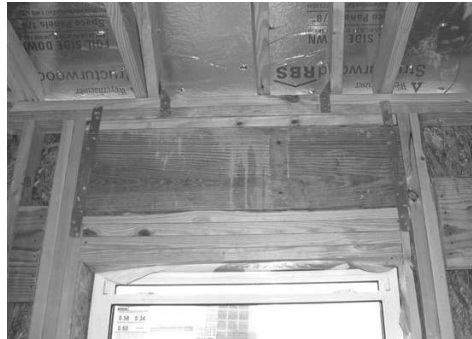
Figure 17. The straps nailed to the window framing studs and to the top plate provide continuity to resist the uplift forces over the window opening.
