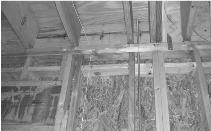
Figure 15. The continuity to resist uplift forces in this critical area between floors is developed through the OSB panels that straddle the first and second floors with their edges nailed and glued to the solid blocking provided near the top of the first floor level. The threaded rod extends through the top plate of the first floor wall to anchor the top plate of the second floor wall to additionally resist uplift forces.
