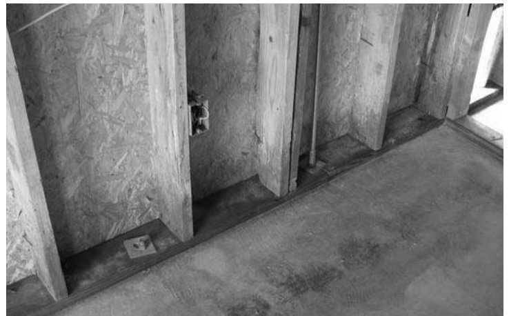
Figure 12. The bottom plate anchor bolts are typically placed at 30" on centers.
