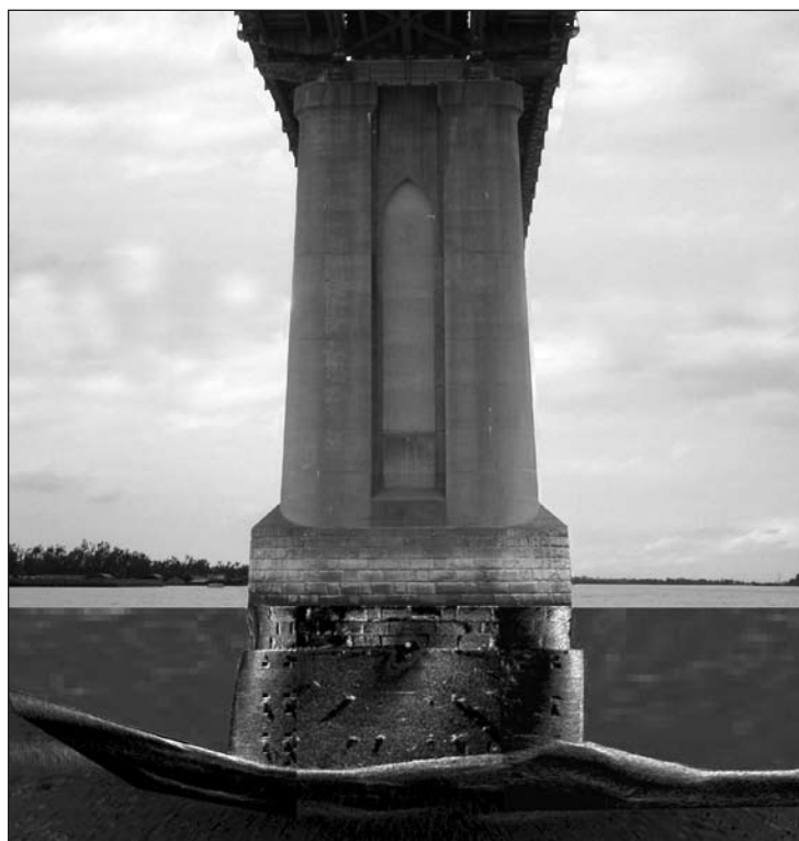
Figure 8. Visualization of the longitudinal pier alignment plane, Huey P. Long Bridge in New Orleans, LA
