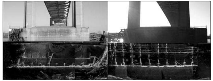
Figure 4 - Bridge Pier Fender Damage assessment
