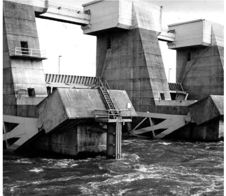
Figure 2 – Sediment sampling installation by pumping a mixture of sediment and water from a highly turbulent flow area of the Auxiliary structure at the Old River Control Complex (ref: 2).
