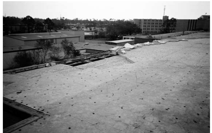
Figure 4. Three story building damaged during Hurricane Rita with loss of roof cover and roof deck.
