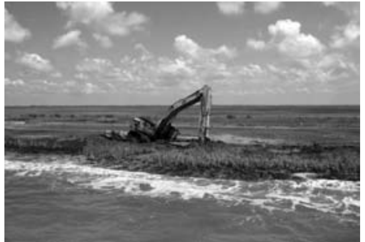
Figure 14. Track hoe on timber mats partially submerged in soft soils.
