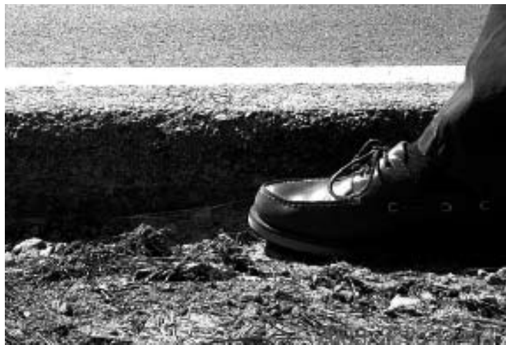
Sharp, steep pavement edge drop-offs can contribute to crashes.
