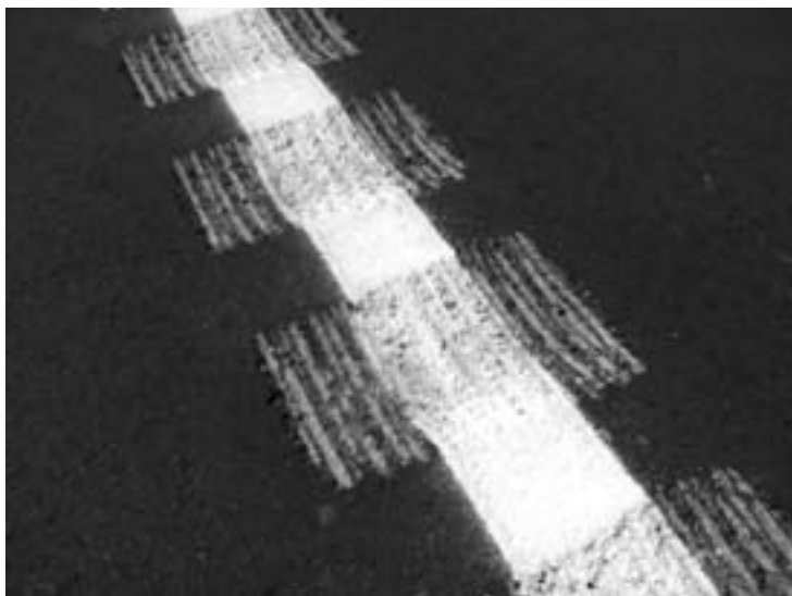
Four-inch edge line rumble stripe placement on a rural highway
