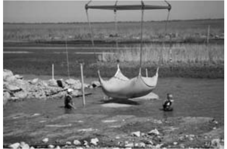
Figure 13. Geotextile bags being lowered into place.
