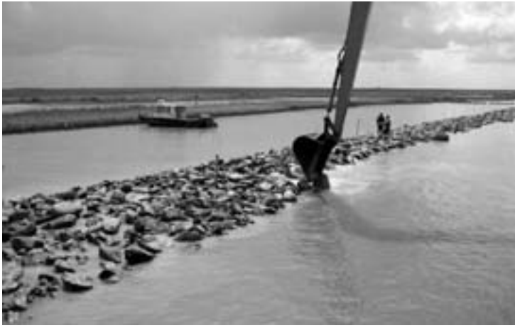
Figure 10. Placing graded riprap along Reef Breakwater.
