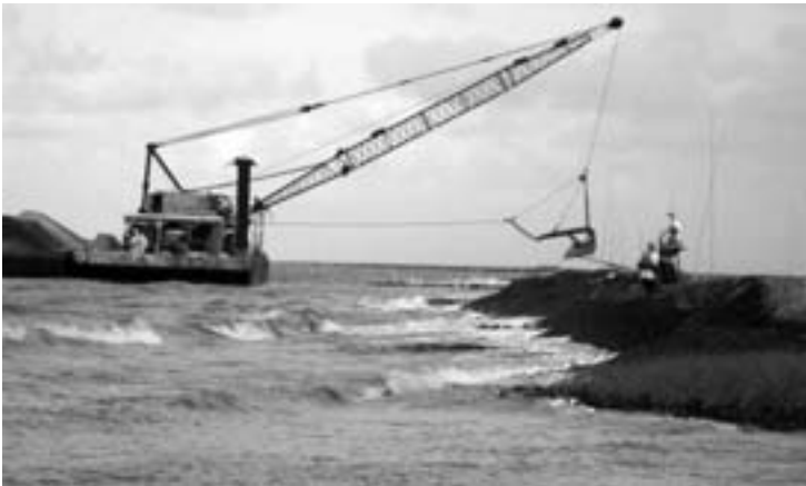
Figure 11. Placing gravel as Beach Fill.
