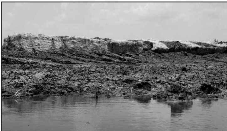
Figure 7. Using hay bales to bring a containment dike up to grade.
