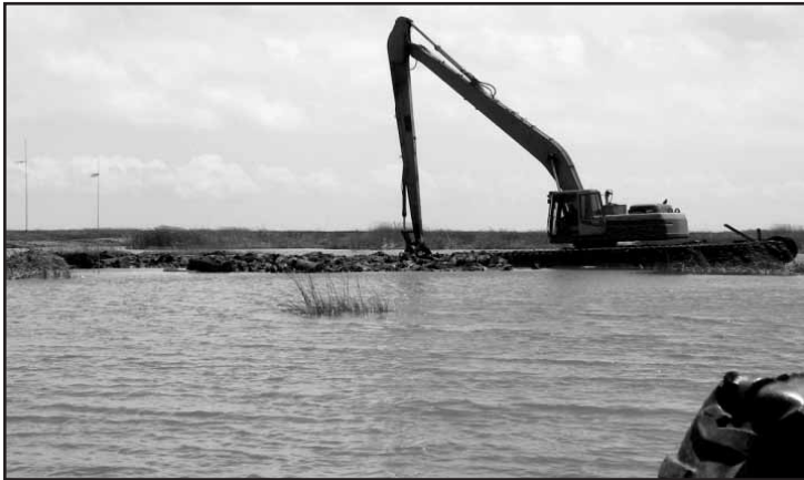
Figure 6. Marsh buggy constructing containment dikes.
