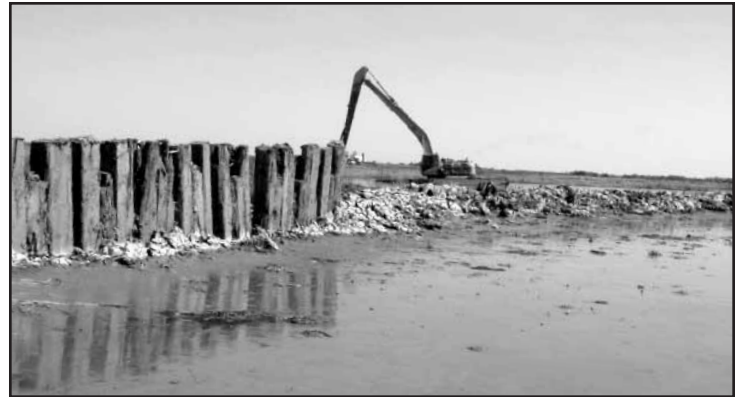
Figure 8. Using timber mats to close a containment dike breach.
