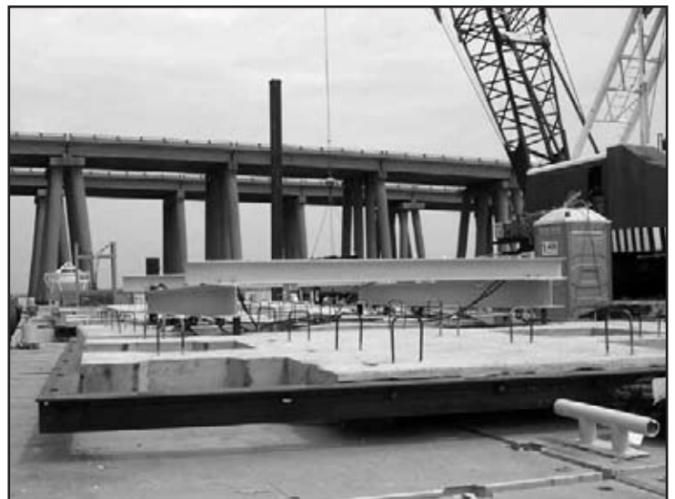
Figure 7. Permanent precast footing form
