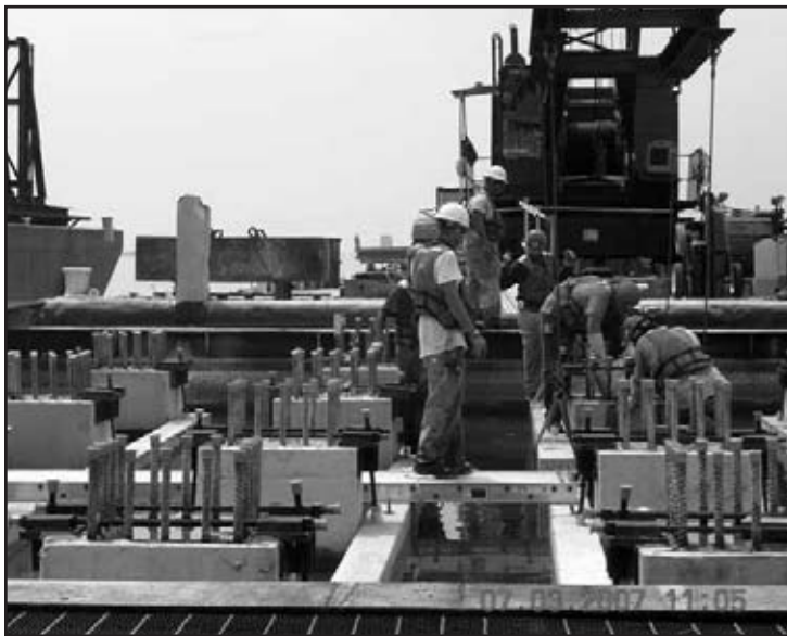
Figure 5. Moment connection for footing piles
