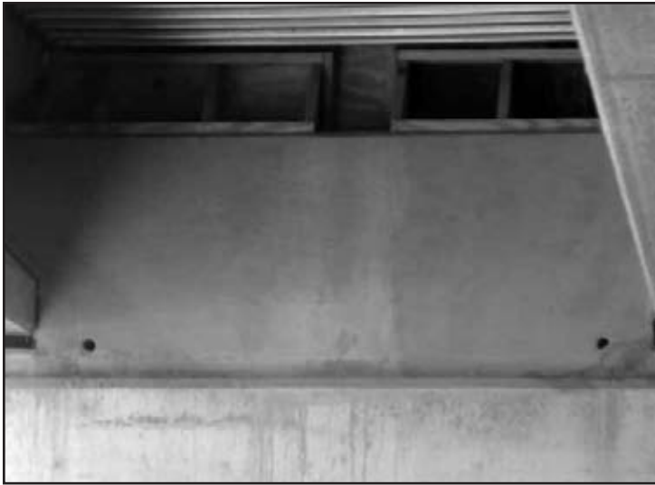
Figure 8. Type III end diaphragm
