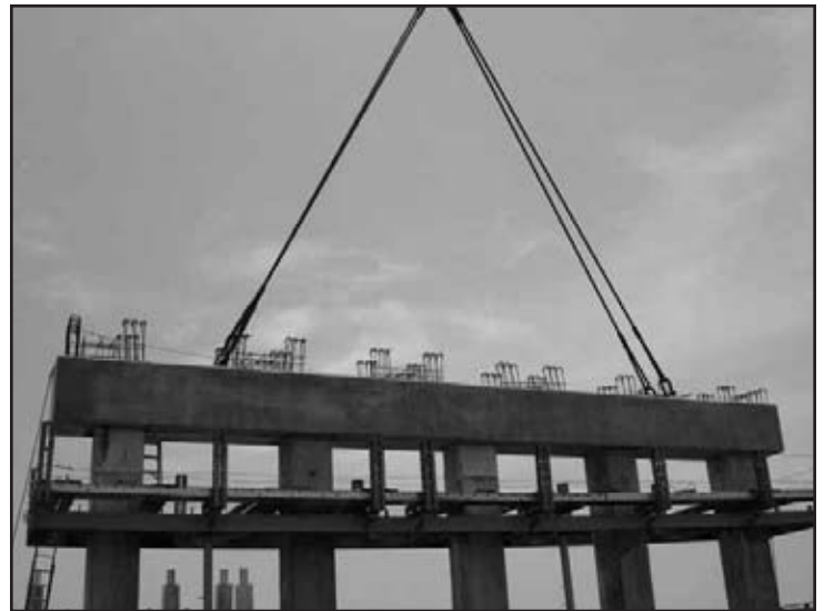
Figure 6. Precast concrete caps
