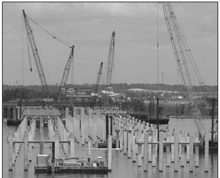
Figure 4. Precast prestressed concrete piles 36-inch
