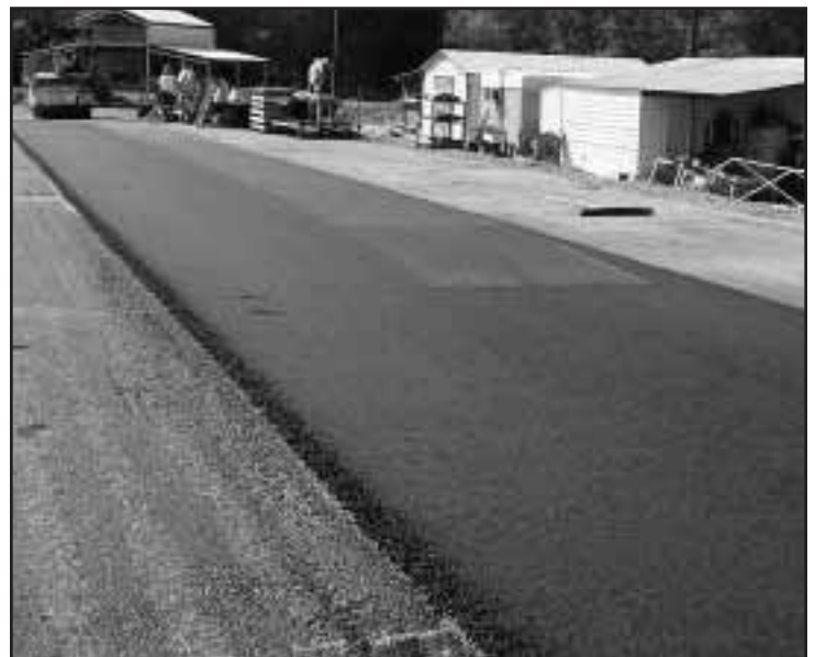
Figure 7 - Conventional tack coat application and paving equipment over an existing HMA pavement surface
