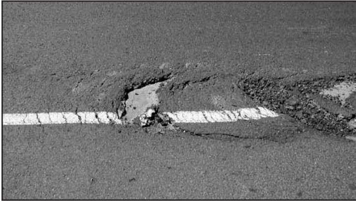
Figure 1 - Delamination appears as crescent-shaped cracks
