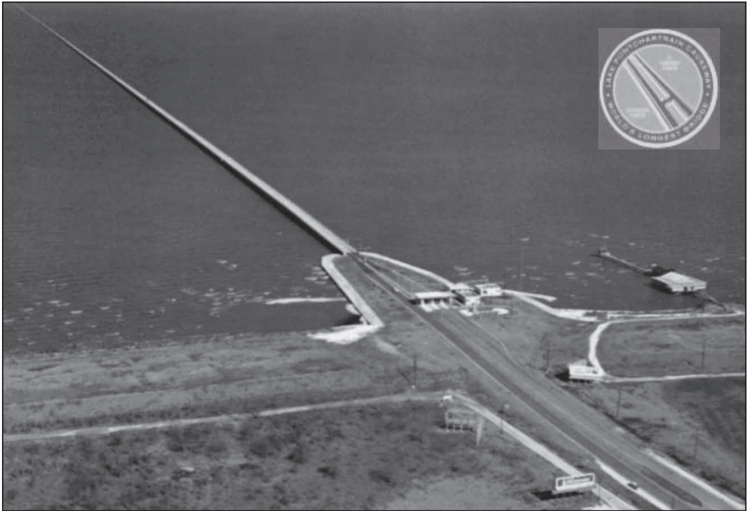
The Lake Pontchartrain Causeway Bridge 1956-2012
