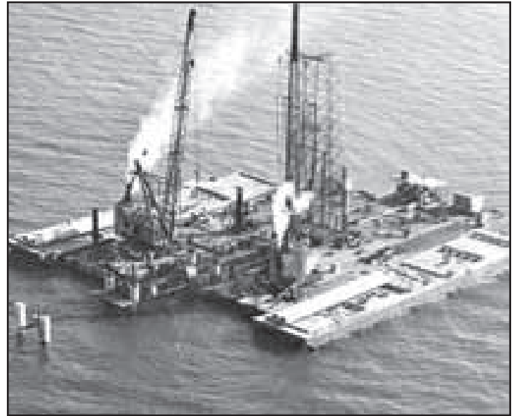
Transporting components via barges
