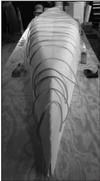
This is the concrete Canoe form for this year's canoe; we are looking forward to pouring in the next few weeks
