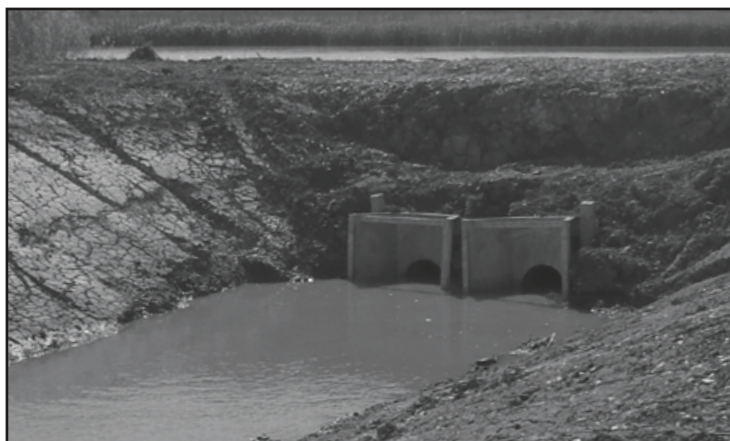
Figure 3. View of Culverts From Within Marsh Creation Area
