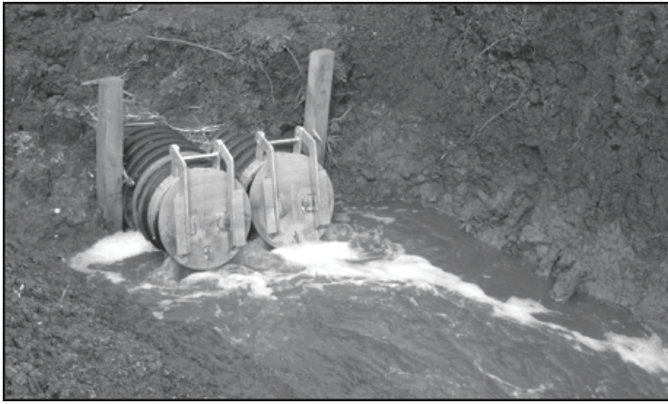
Figure 4. View of Culverts From Outside of Marsh Creation Area
