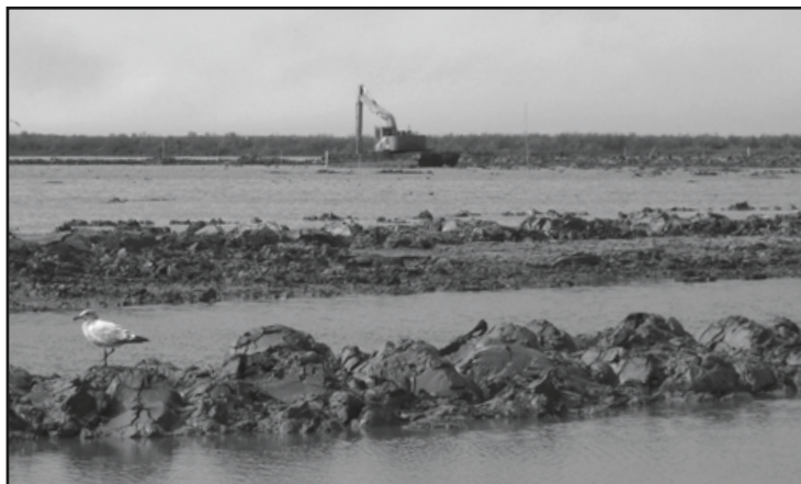
Figure 2. Temporary Internal Training Berms and Tidal Channel
