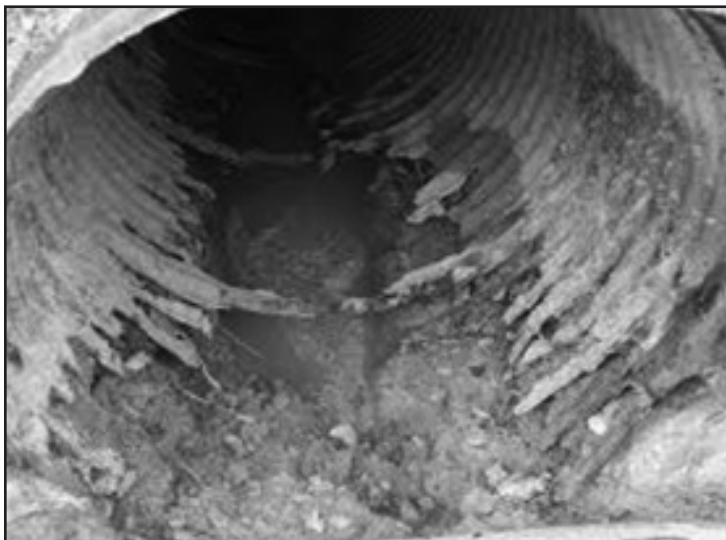
Deteriorated culvert
