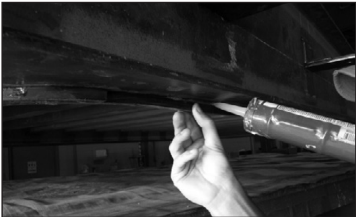
TTC’s Small SCTA – positioning of the seal and bladder
