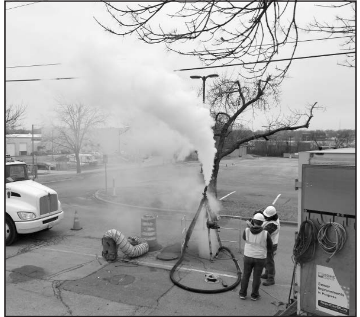
Vertical exhaust steam curing in St. Louis, MO.
