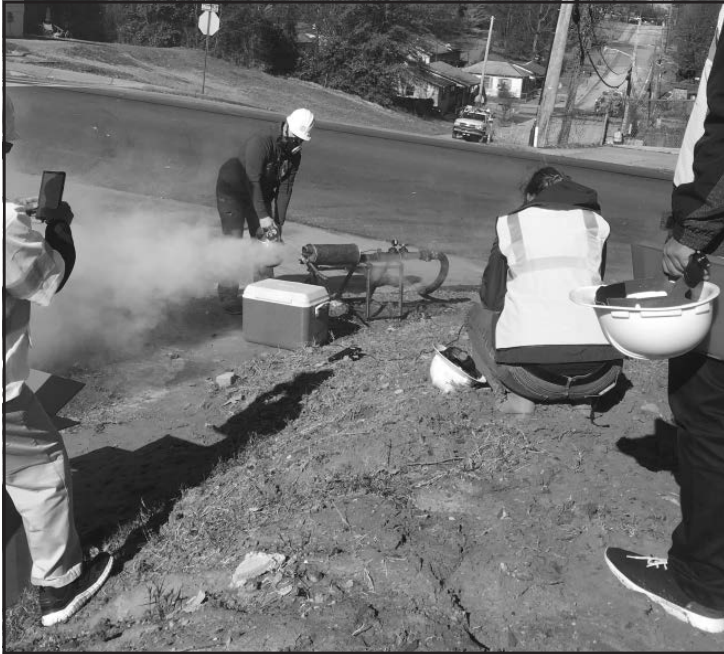
Horizontal exhaust steam curing in Shreveport, LA.
