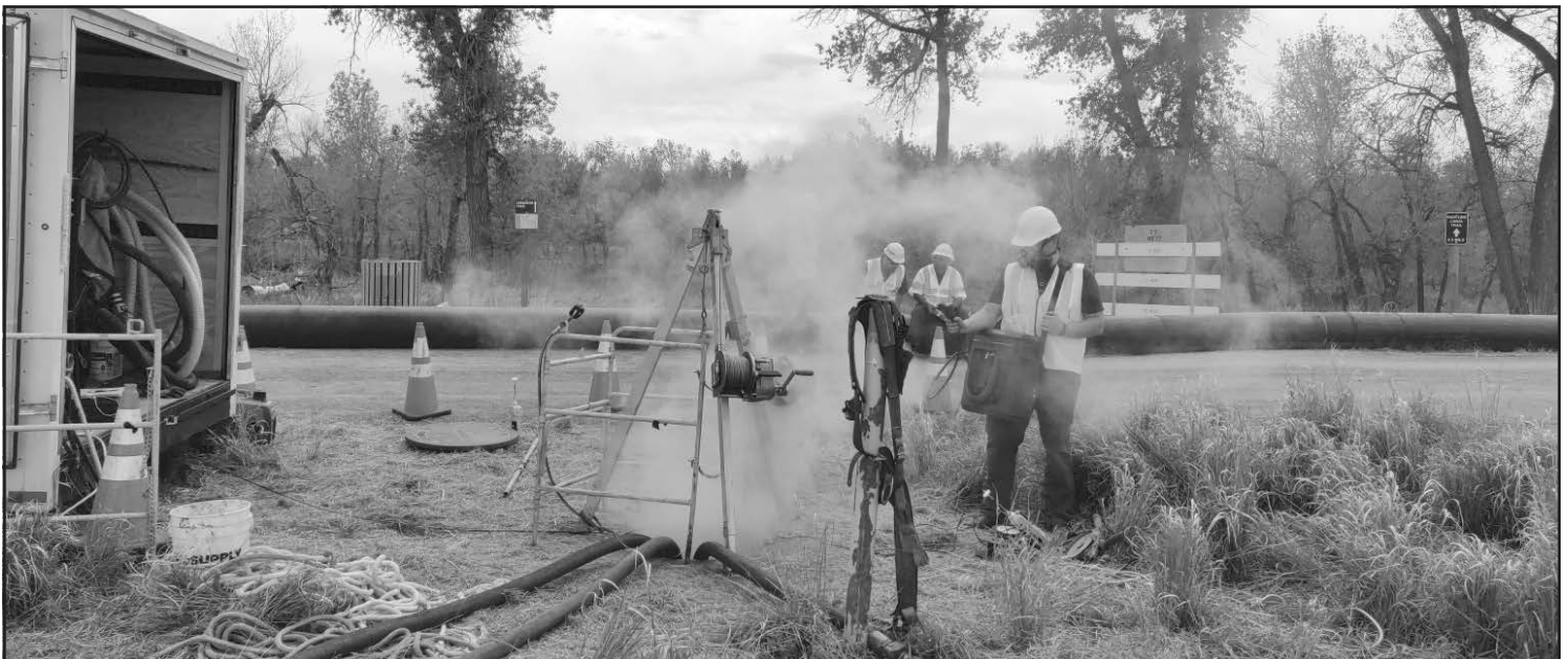
Large-diameter steam curing in Aurora, CO.
