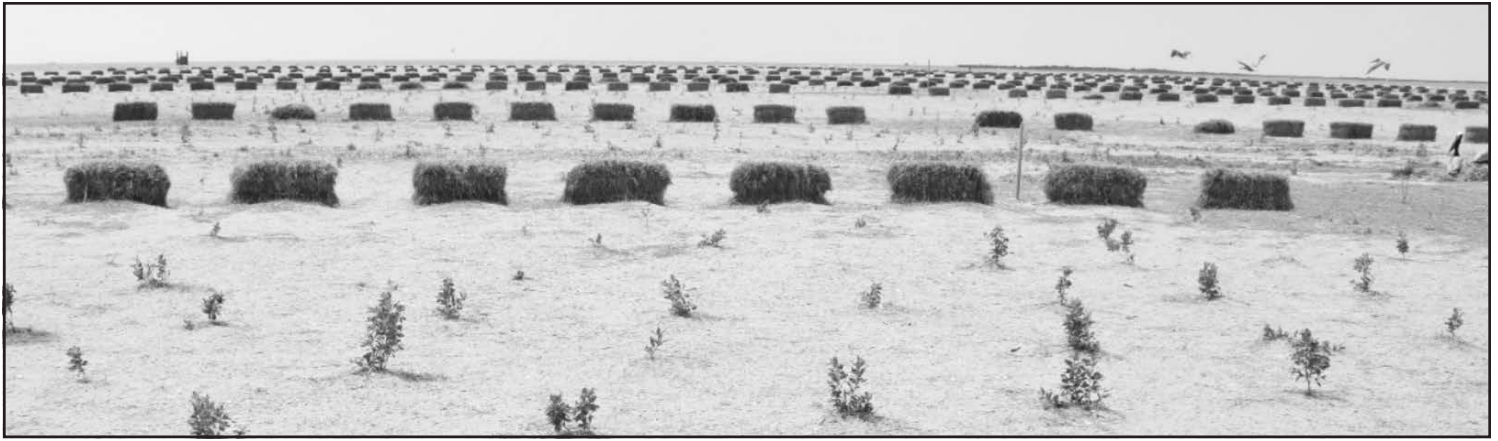
Figure 3: Installed Hay Bales and Vegetative Plantings on Queen Bess Island (Photo credit: LDWF)
