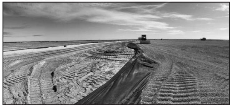
Figure 2: Construction Crews Installing the Limestone Material in Cell 3
