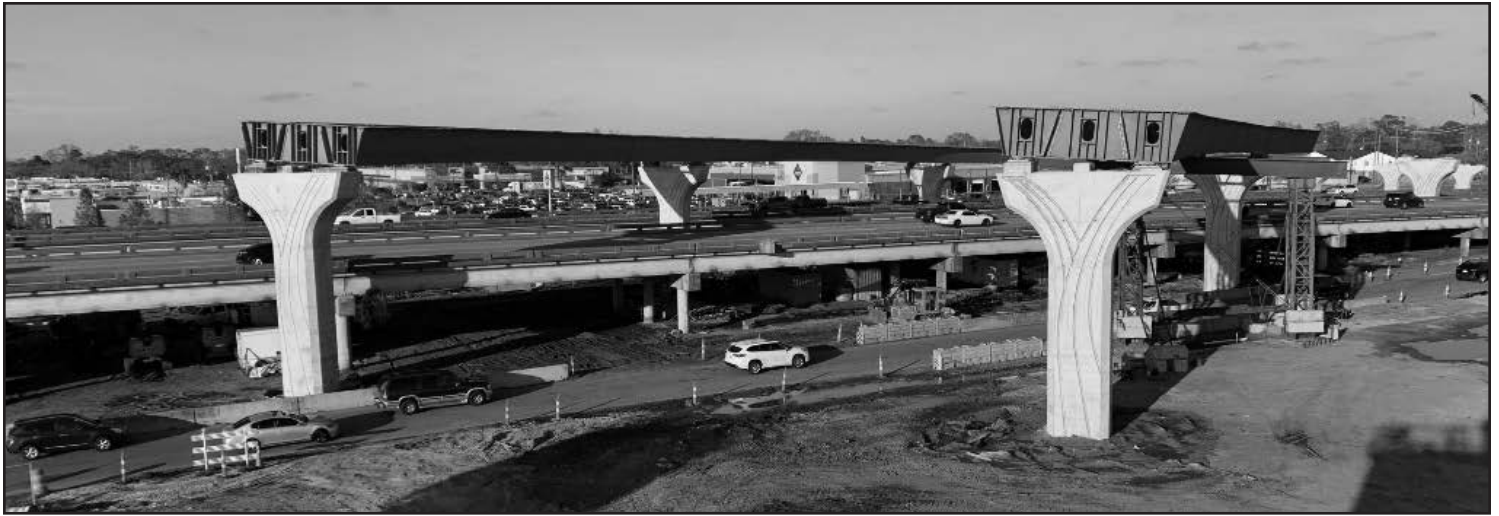
Figure 7 - Steel Tub Girders Erected over I-10
