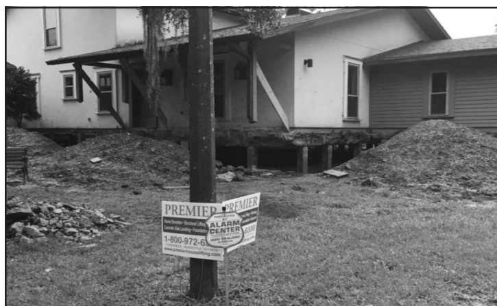
Figure 1 A House in Baton Rouge, LA Being Raised Following Repeated Flooding
