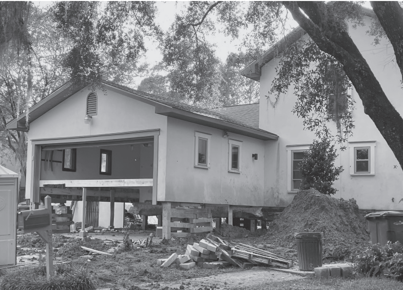
Baton Rouge, LA – House Being Elevated Following Repeated Flooding
