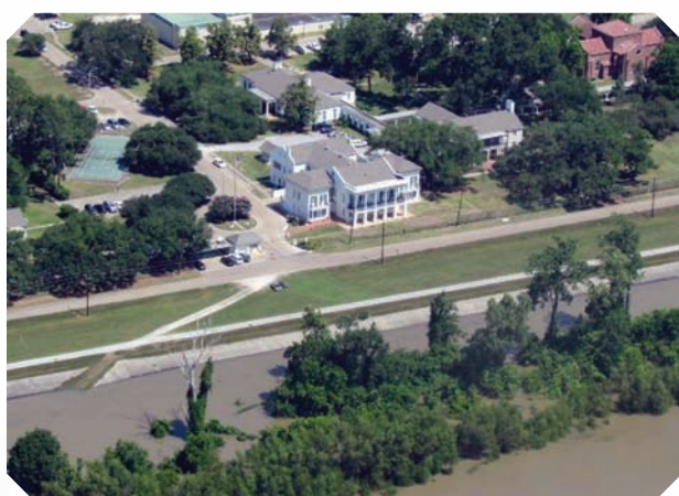
FIGURE 3: A MISSISSIPPI RIVER LEVEE WITH SLOPE PAVING PERFORMING DURING HIGH WATER IN 2011
