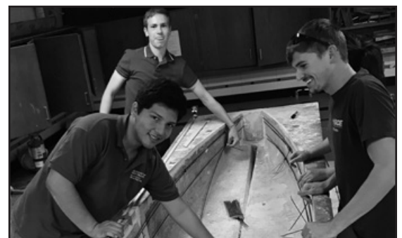
Preparing Mold for Concrete Pour in Concrete Lab at UNO (from left to right: Francisco Avelar, Homero Toledo, and Spencer Marston)
