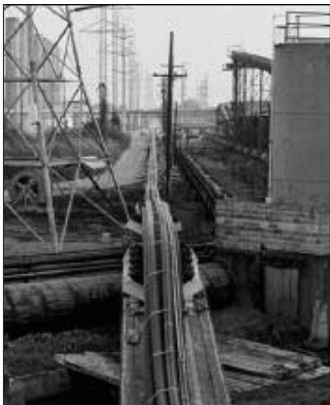
Figure 12. View looking north away from the river of backstring ready for pullback operations.
