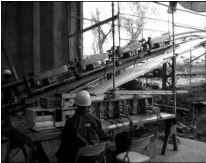
Figure 20. The cable haulers or caterpillars located near the entrance of the cable to the duct in the termination structure on the east bank.
