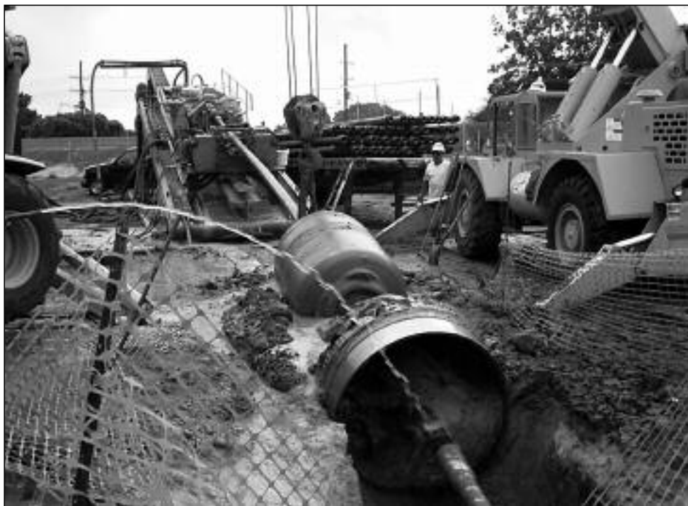
Figure 11. 48" swab followed by the 54" reamer being pulled through the hole as it emerges at the drilling rig.
