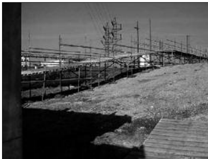
Figure 19. Ramp to support and guide the cable from its pipe to the crown of the levee on the west bank.
