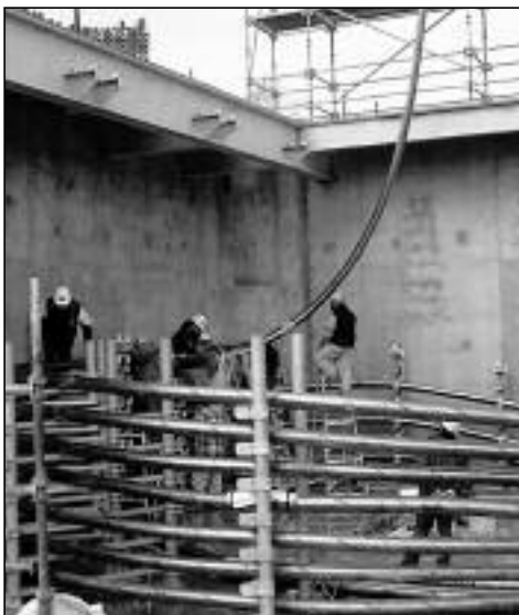
Figure 21. A cable is being lowered by a crane and coiled or racked on the coil support structure.
