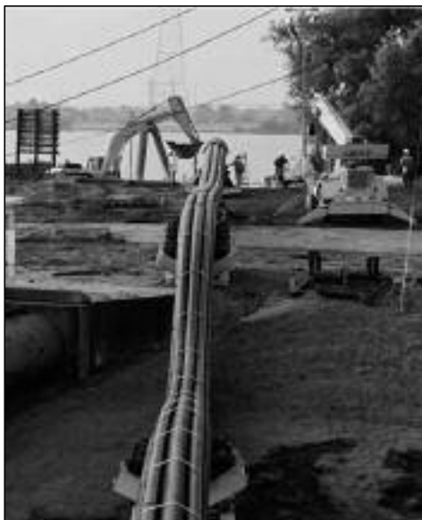
Figure 13. View looking south toward the river of backstring ready for pullback operations.
