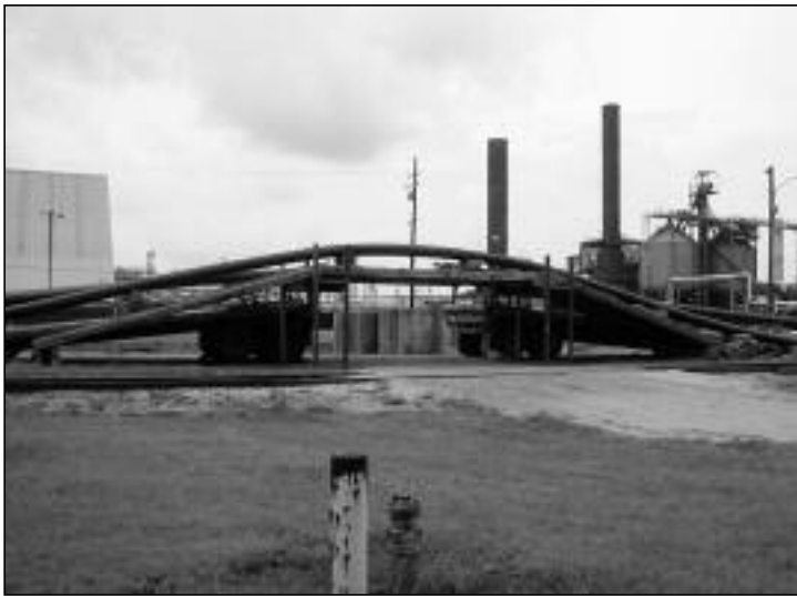
Figure 5. Temporary bridge for the backstring to provide access to the plant facilities on either side of the backstring fabrication site.
