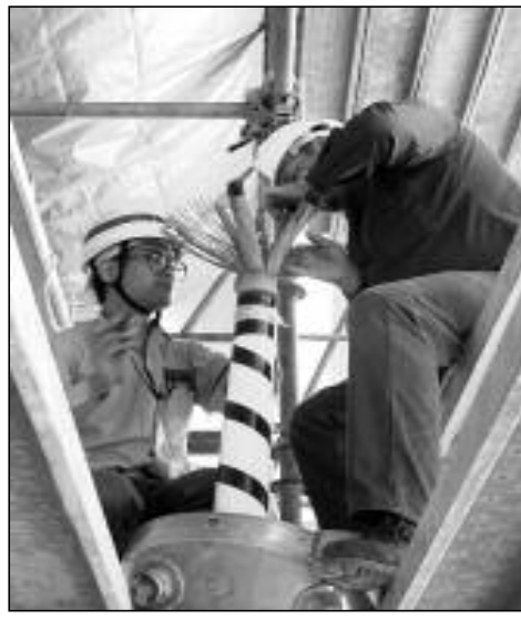
Figure 23. The strands at the end of a cable are being manually splayed in preparation for sandblasting to remove the enamel insulation.
