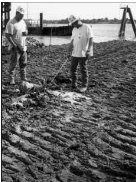
Figure 10. Drill emerges 4" from the planned exit point. The point of the delta loop is visible to the right of the exit point as are the electrical wires that lead to the 2 dolphins — one shown in the background.
