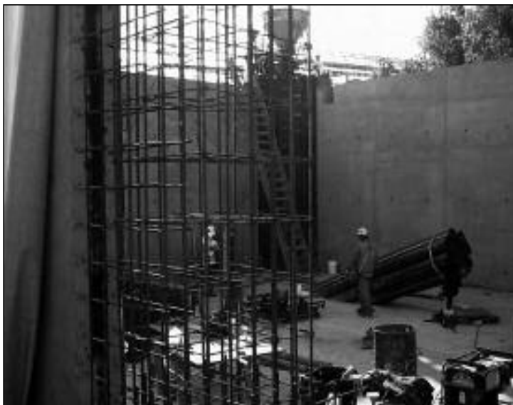
Figure 16. Construction of a termination structure showing the end of the duct entering through the floor.
