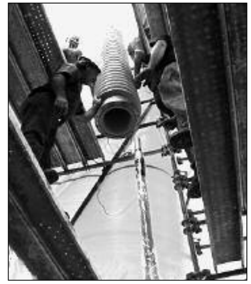
Figure 24. A termination assembly is being lowered to attach it to a sandblasted and reworked cable end and complete the termination.
