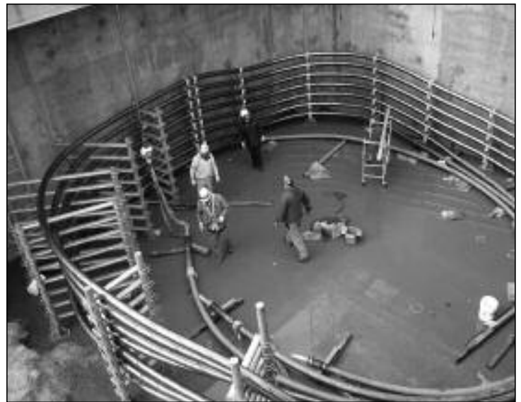
Figure 22. The cable coil support structure inside a termination structure.
