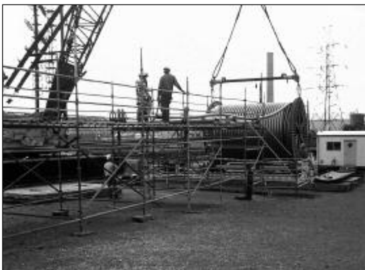
Figure 18. Ramp to support and guide the cable into its pipe from the reel mounted on the handler on the east bank.
