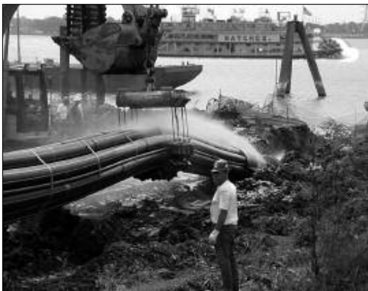
Figure 14. Backstring on the east bank batture at the beginning of the pullback operation showing the 12-pipe duct bundle strapped with stainless steel bands.
