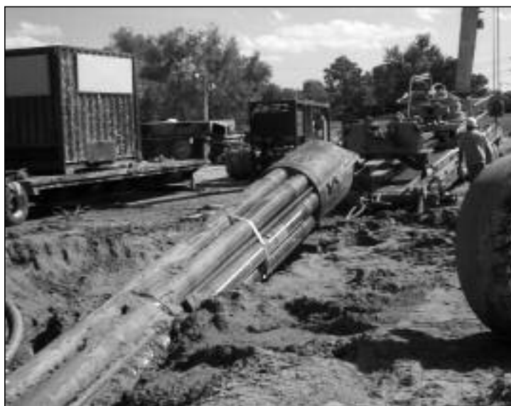
Figure 15. Backstring on the west bank batture at the end of the pullback operation showing the 12-pipe duct attached to the pulling head.
