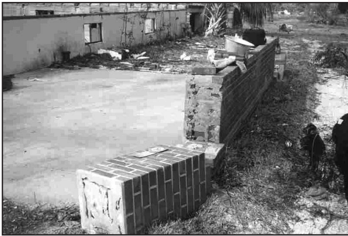
Figure 9. The carport canopy supports at each end of its low wall were lifted and fell away from the wall (sketch number 11).
