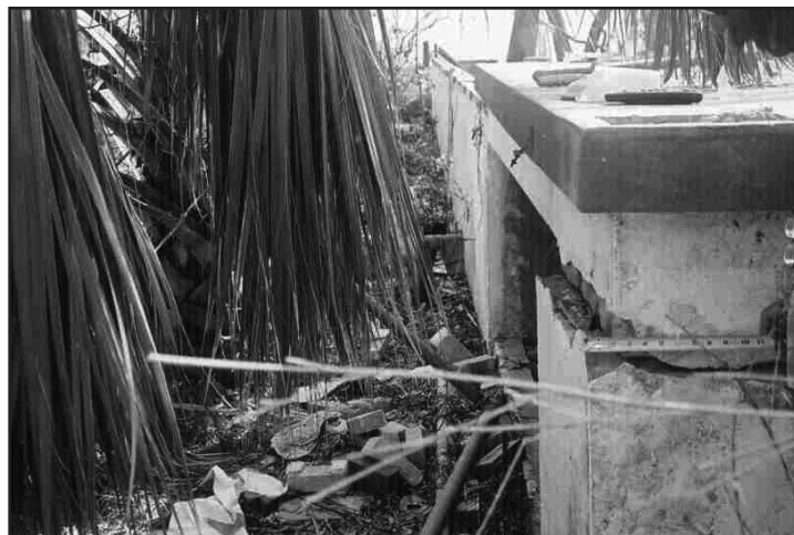
Figure 4. Concrete deck slab is broken from its support and it has moved about 2 1/2" to the west (sketch number 3).
