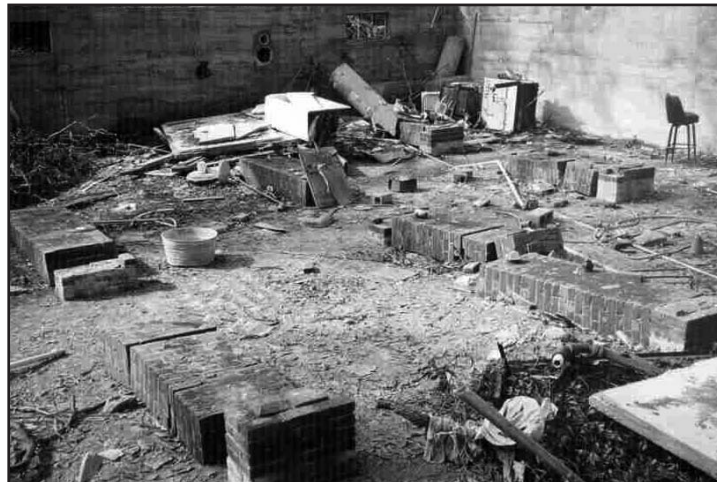
Figure 6. The brick pilasters supported on the basement floor slab fell to the west (sketch number 6). The pilasters together with the basement perimeter walls supported the structure at the first floor level.
