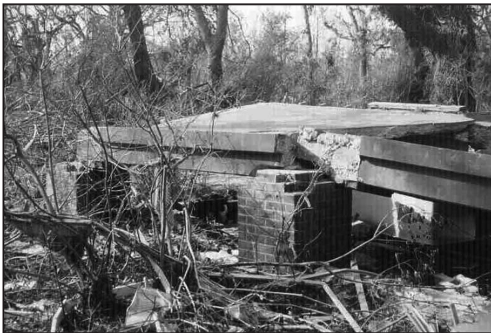
Figure 14. The continuous concrete edge beam supporting the concrete deck on the south side of the residence and spanning between the brick pilasters was cracked and damaged (sketch number 14).
