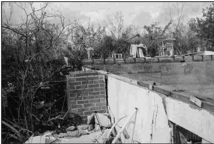
Figure 7. The fireplace was detached from the building and was inclined to the west (sketch number 9).
