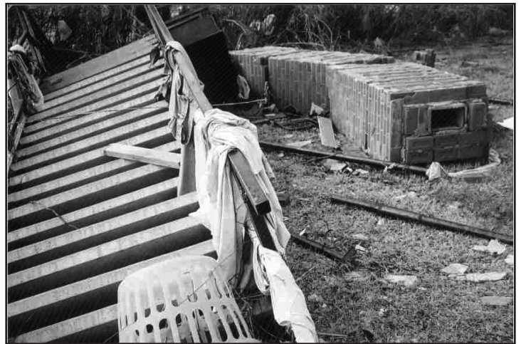
Figure 8. The steel fire escape stair and the chimney located on the west side of the residence fell to the west (sketch number 10).
