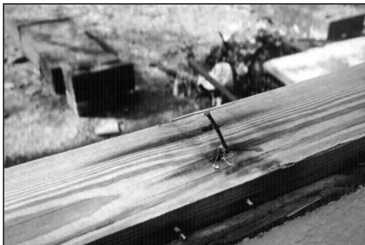
Figure 5. An example of a toenail that attached a stud to the remaining sill plate is typically bent to the west (sketch number 4).
