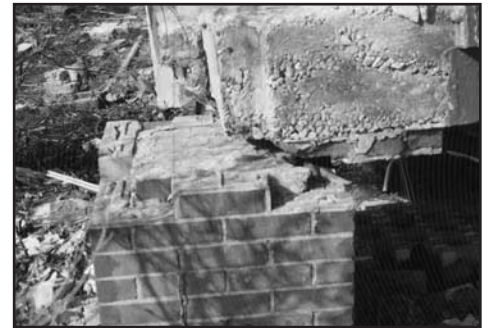
Figure 13. The concrete deck slab at the south-east corner of the residence was detached from its support and displaced 10" to 14" to the north (sketch number 12).
