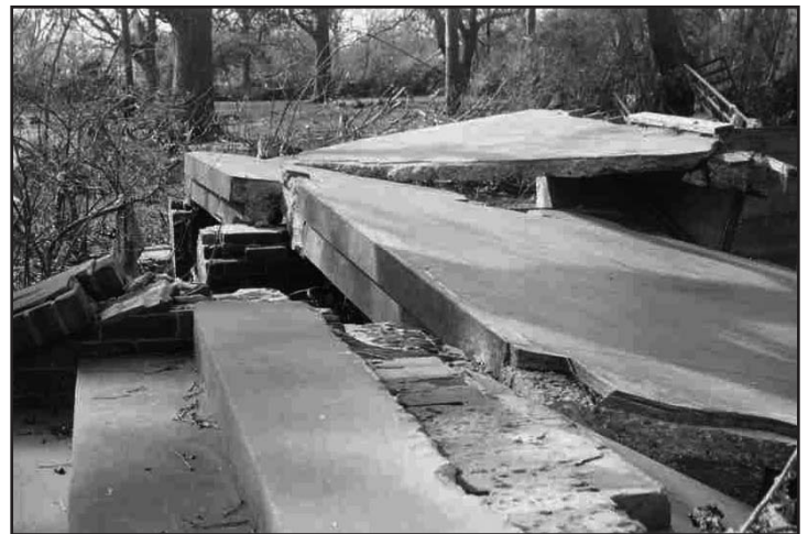
Figure 12. The concrete deck slab on the south (front) side of the residence was cracked, separated into segments and displaced to the north (sketch number 13).
