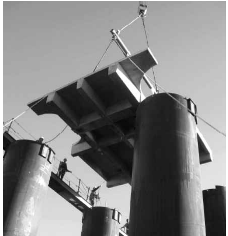
Figure 3. East Pier, Soffit Panels Erected
