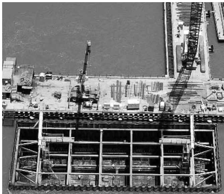
East Cofferdam Upon Completion of Lowering 47 feet
