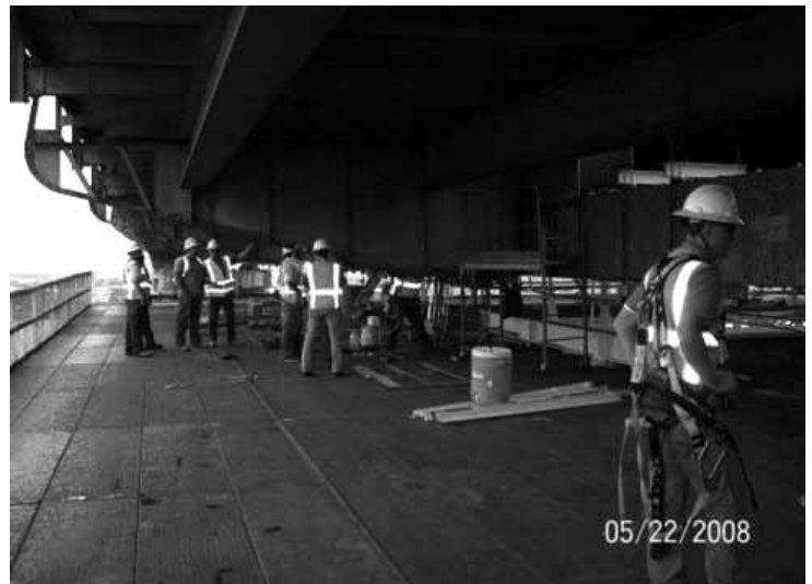
Figure 12 – Work Platform Under Bridge
