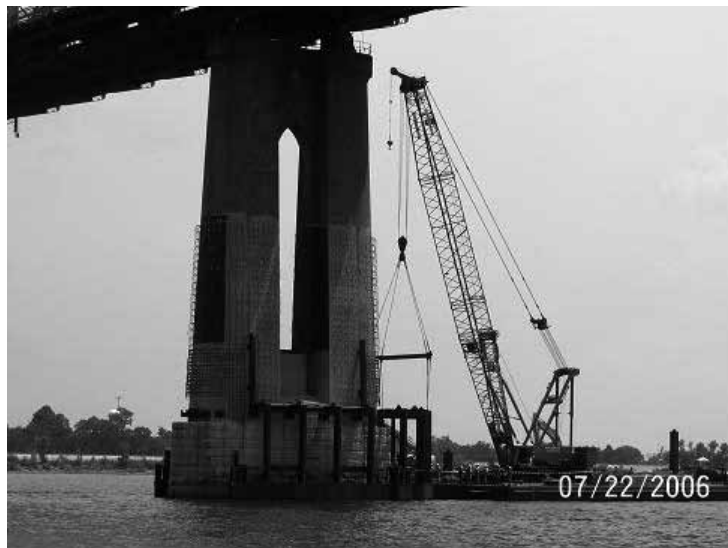
Figure 8 – Erection of Pier Cofferdam
