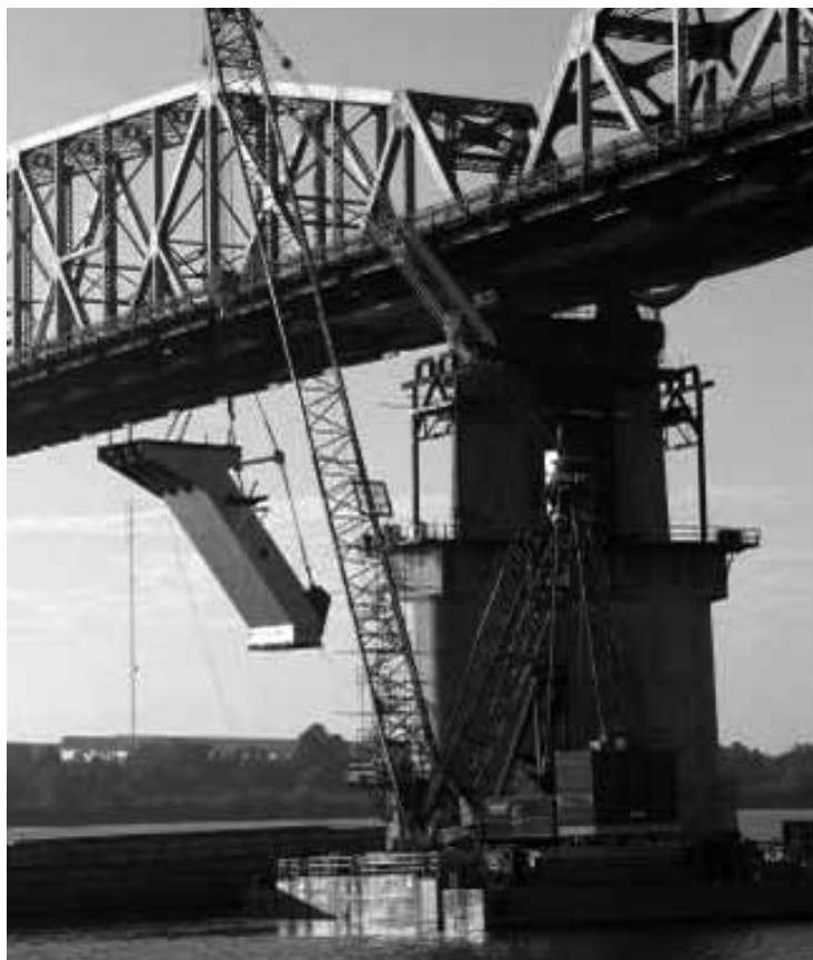
Figure 9 – Erection of Diagonal Strut
