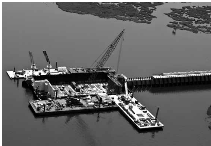
An aerial view of the bypass gate cofferdam and abutments
