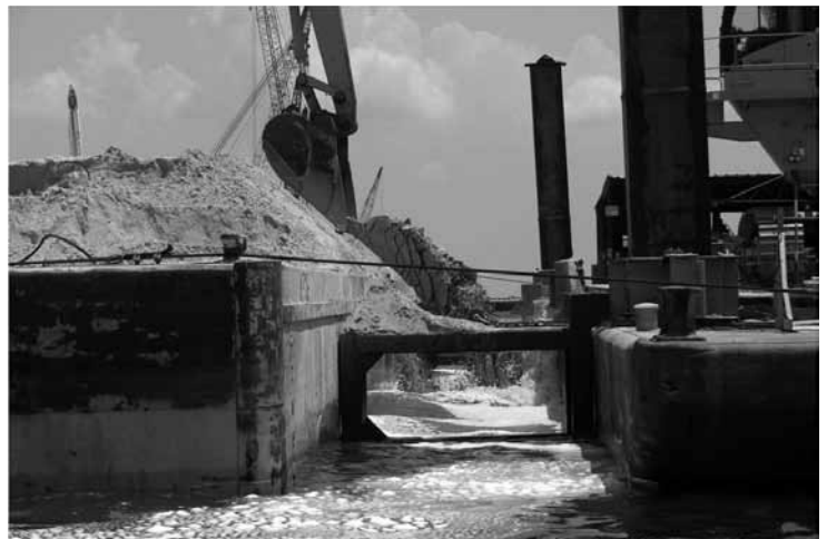
Crews filled the de-authorized MRGO to raise its bottom elevation before driving piles in the channel
