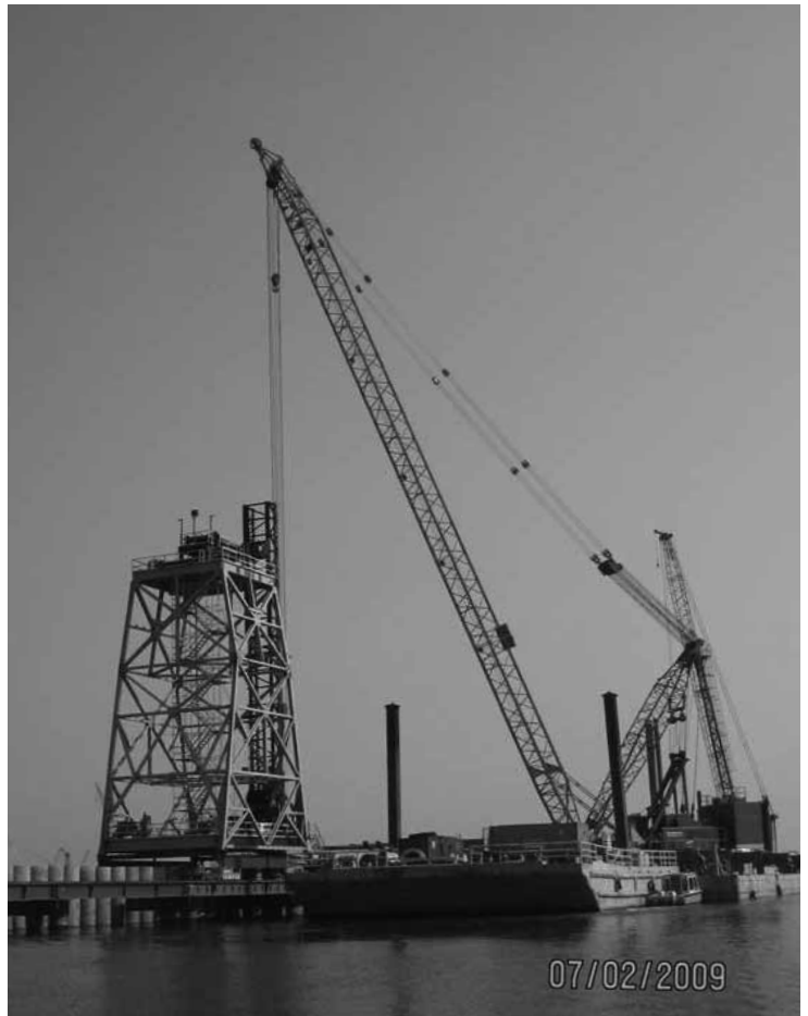
The Whirley Tower (yellow structure) served as the leads and the template for the soldier piles on the north heading
