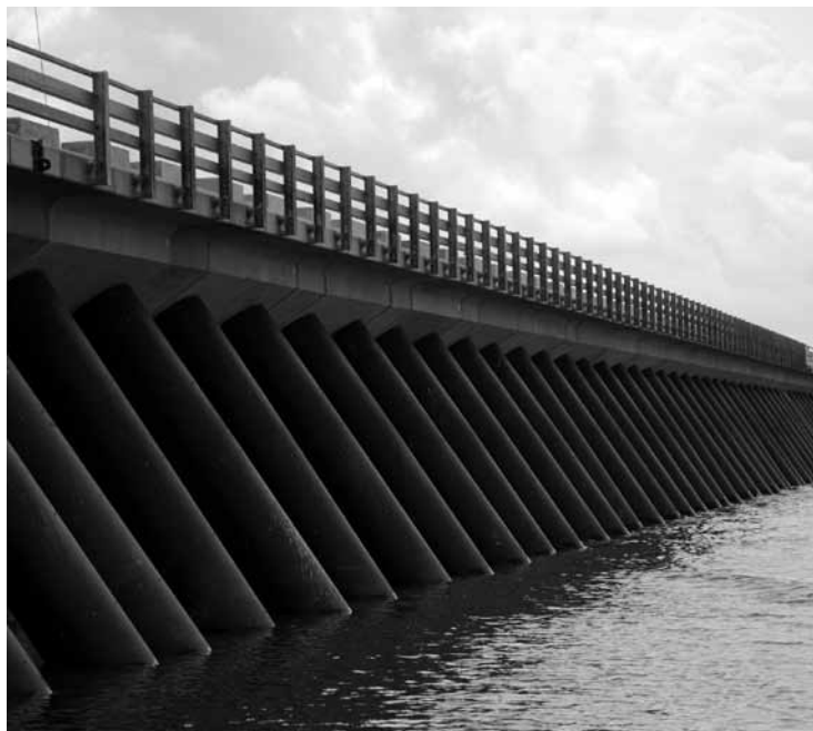
Angled steel batter piles line the protected side of the surge barrier wall Credit: USACE Photo by Paul Floro
