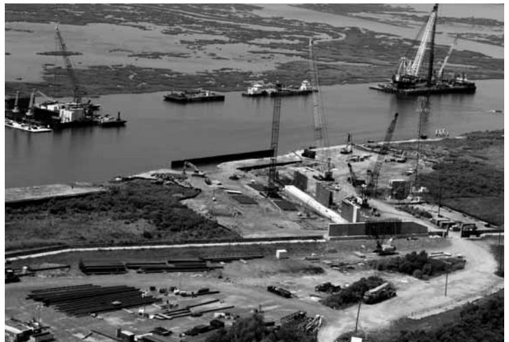
An overhead view of construction of the north T-wall tie-in, with the bypass gate cofferdam in the top left of the photo
