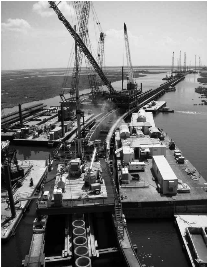
The trestle track provided a level surface for rigs to move along the barrier wall
