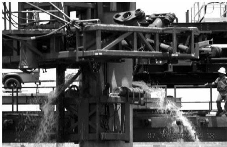
As soldier piles were driven deep into the water and mud, weep holes along the side of the piles allowed for drainage to relieve pressure
