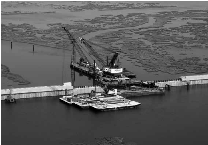
Crews construct a cofferdam at the Bayou Bienvenue gate
