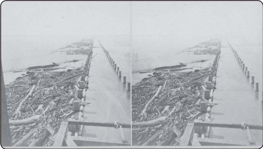
View of piles for jetty taken from the pile driver, showing Port Eads in the distance.
