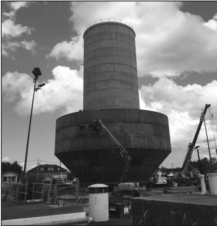
Figure 7- Steel Tank Onsite Fabrication
