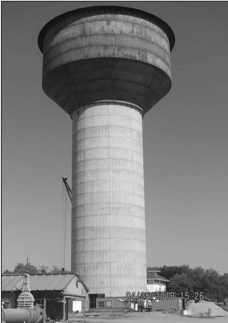
Figure 8- Installed Steel Tank for Panola Water Tower
