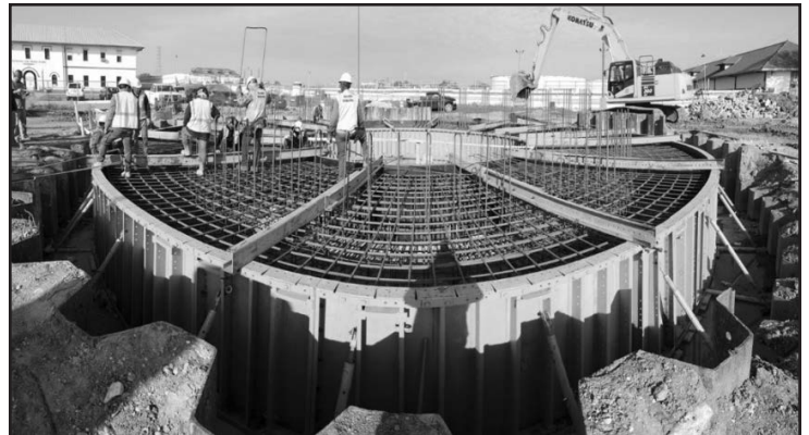
Figure 5 – Claiborne Water Tower Foundation
