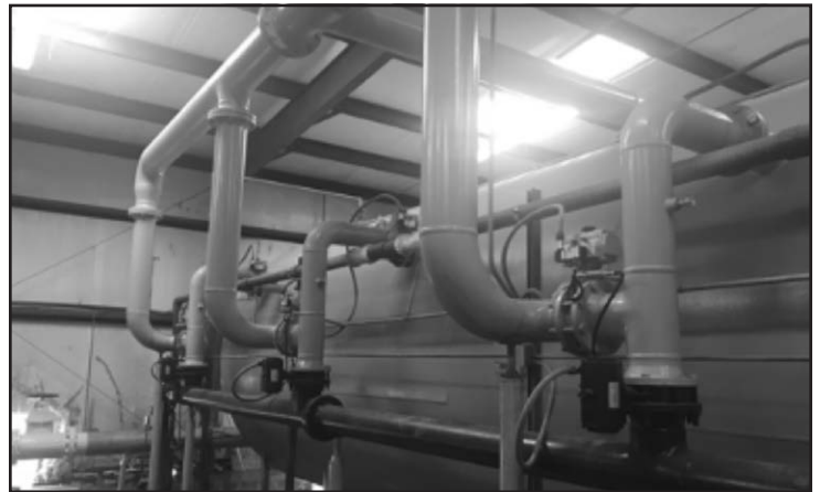
New pressure filter at the water treatment plant
