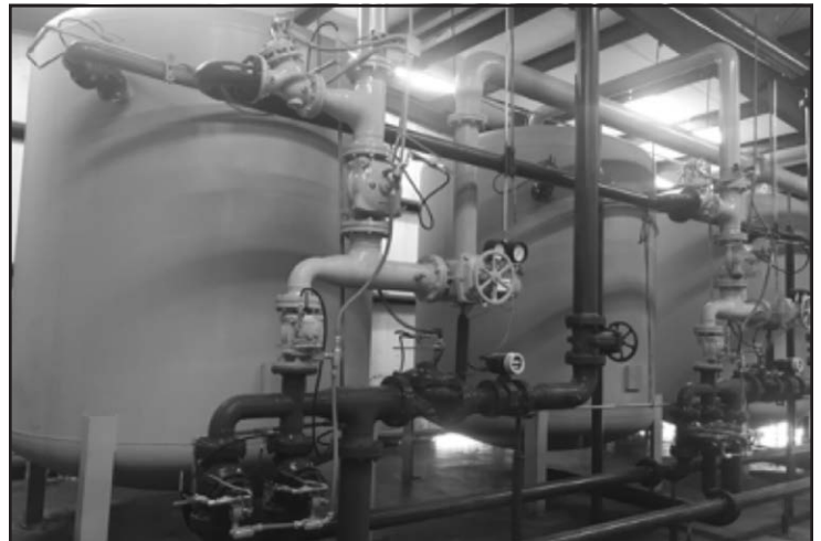
New softener bank at the water treatment plant
