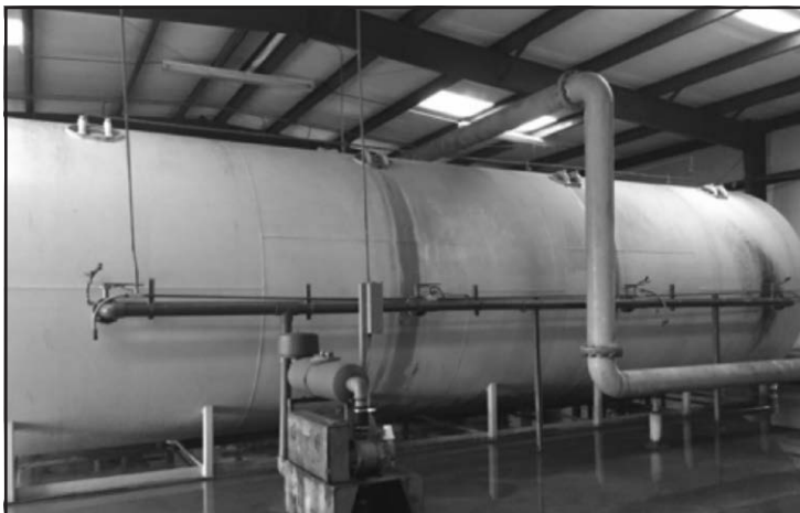
Existing pressure filter at the Town of Saint Joseph's old water treatment plant
