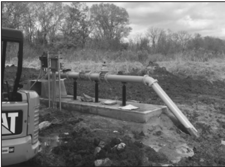
Installation of the new water well
