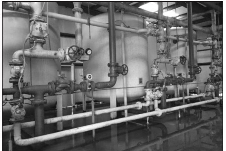
Existing softener bank at the Town of Saint Joseph's old water treatment plant
