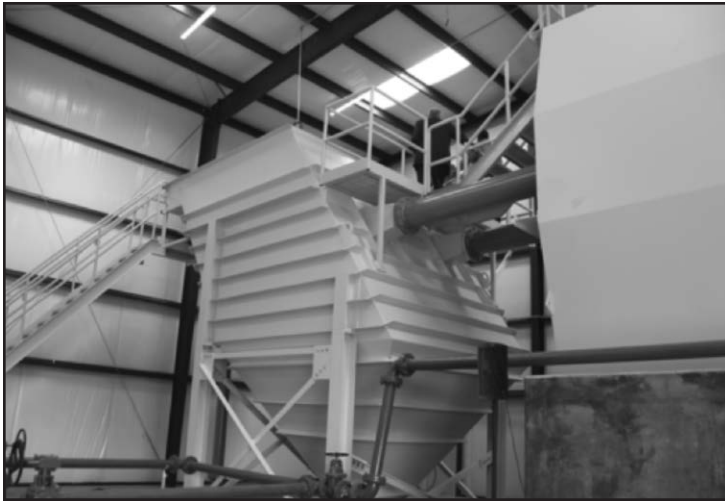
The AIS system consists of a reactor basin (aeration, flocculation) and a clarifier, photographed here
