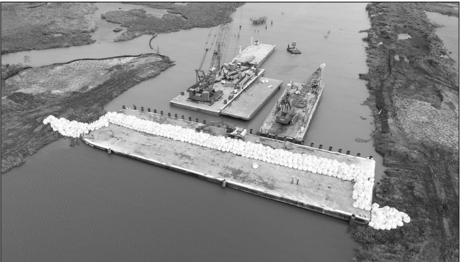
Complete emergency barge closure, Oct 9, 2020
