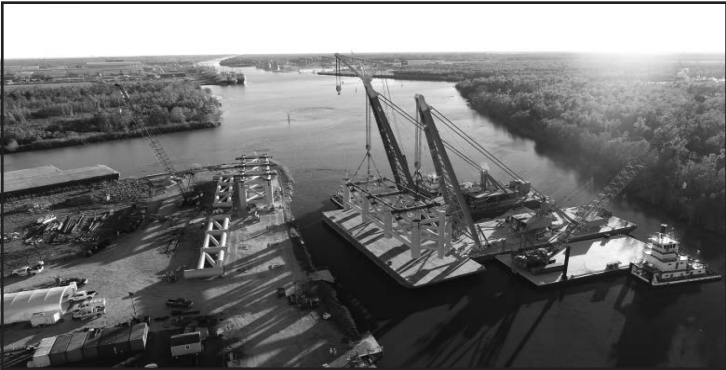
Transport of the Bayou Chene Flood Protection Jacket Structure (1.2 million pounds)
