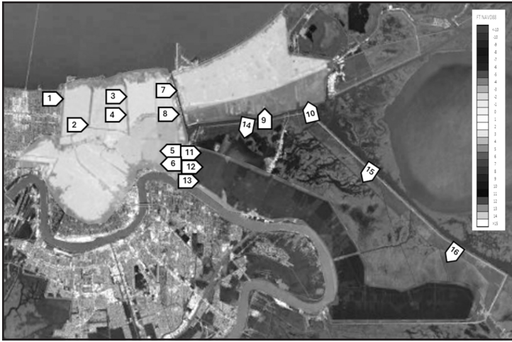
Figure 9. Location of 16 Major Perimeter System Failures During Hurricane Katrina
