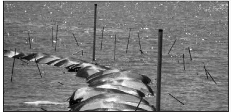
Figure 10: Biloxi Marsh lightweight aggregate filled bags in place
