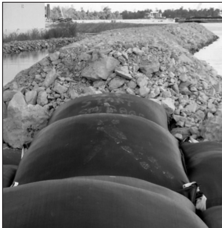
Figure 7: Lightweight aggregate filled geotextile bags before (foreground) and after (background) armoring with riprap
