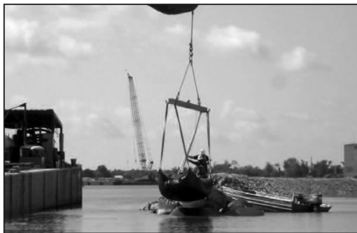
Figure 6: Lightweight aggregate filled geotextile bag placement
