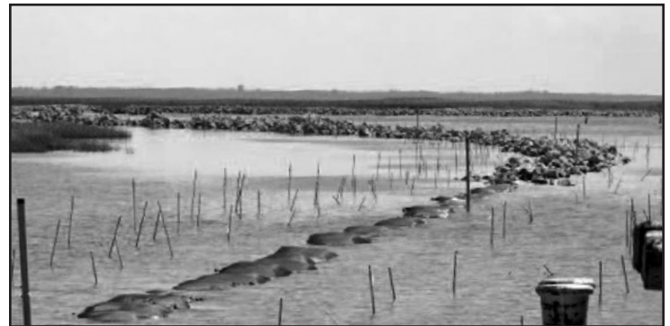
Figure 11: Biloxi Marsh berm before (foreground) and after (background) armoring with riprap
