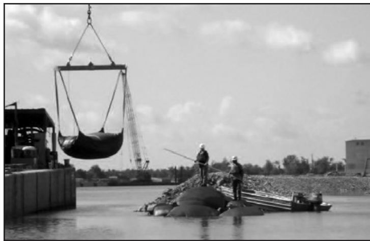
Figure 5: Lightweight aggregate filled geotextile bag lifted from deck barge
